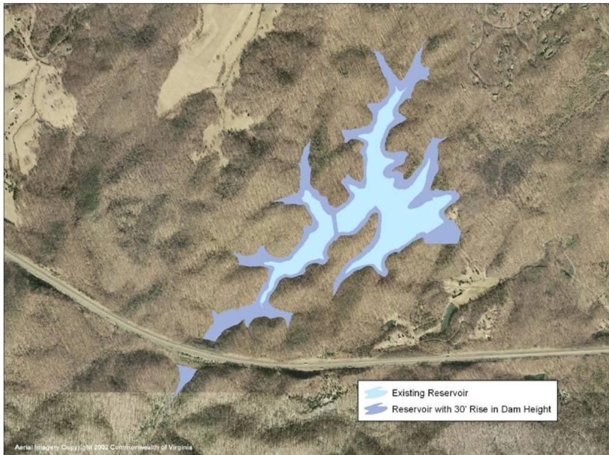
Figure 2. Aerial view of the Ragged Mountain Area showing extent of future inundation. Note that there is no river entering this small watershed. The majority of the water in this pool is presently piped from the Moormans River 14 miles to the west.
